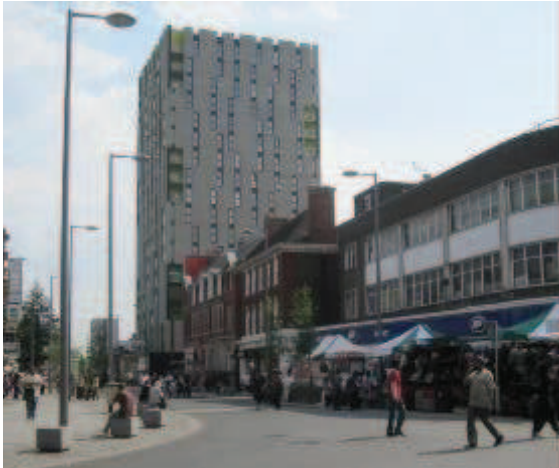
New paving, street furniture and a new road layout to accommodate the new ELT1 at the southern end of Station Parade and Ripple Road.
