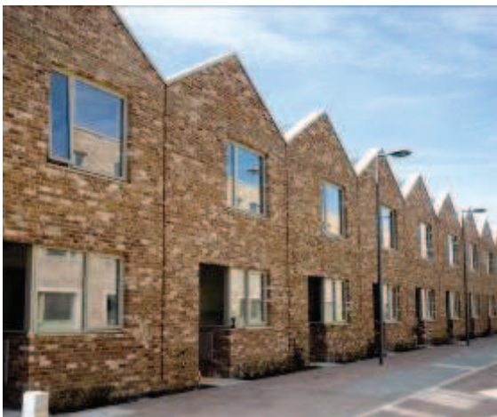
New homes at William Street Quarter present the opportunity to improve pedestrian links to this and surrounding residential areas.
