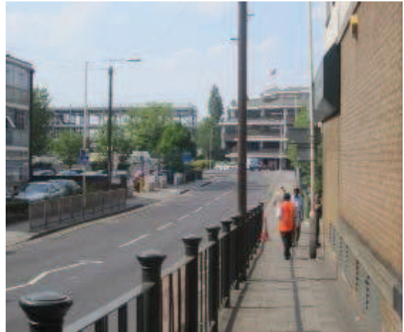
Key walking routes are poorly overlooked, lacking active frontages and natural surveillance.
